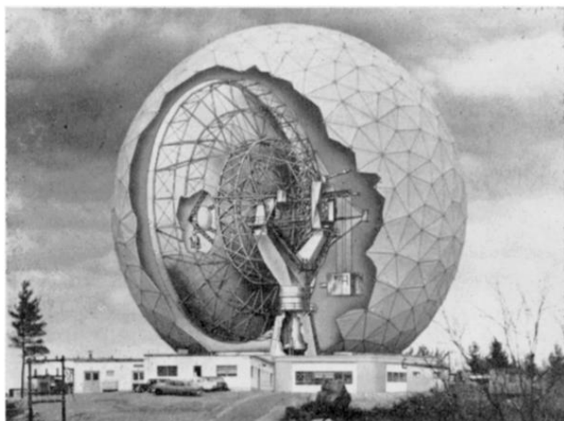
FIG. 2. An artist's sketch of the M.I.T. Haystack radar system, which employs a 120-foot precision parabola mounted inside a 150-foot space frame radome. This antenna operates as a radar at a wave length of 3.8 cm. The radar equipment is housed in a box that is hoisted into a position immediately behind the reflector apex.
